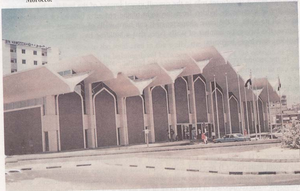
Fig. 5. An example of roof dominated building, full enclosure: Sharja (UAE) Post Office building.
