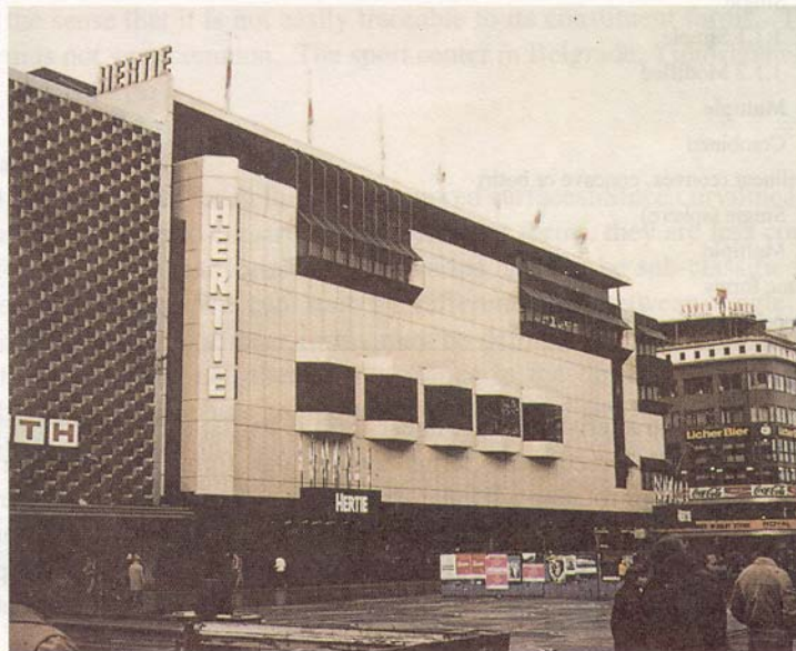
Fig. 11. A commercial building in Frankfurt, Germany. This is an example of a relief wall, where flat areas are contrasted with projections or cavities.
