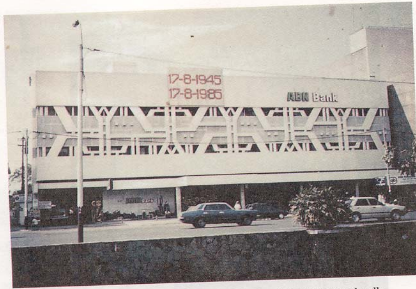
Fig. 12. An example of a wall design utilizing contrast between plain and textured walls.
