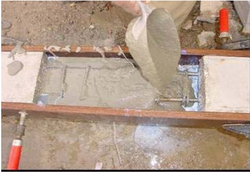
Fig. 2. Application of primer and repair material.
