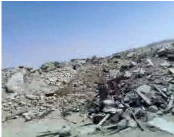
Fig. 5. Industrial cement waste-disposal site S11.
