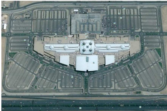
Fig. 11. Google Earth View of a big box shopping mall “Grenada Center” with 4500 parking spaces at the third ring buffer (the outer ring) is a sign of the sprawling development taking place to the north east of Riyadh.
