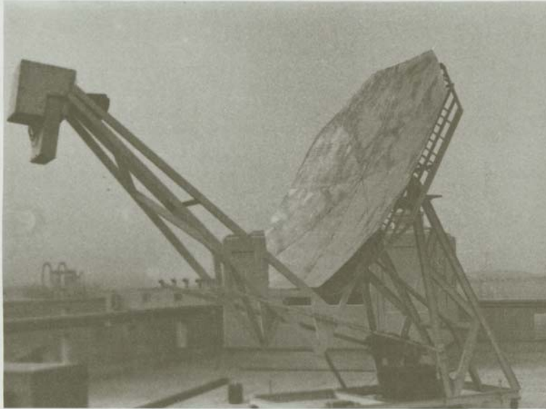
Fig. 5. Offset reflector and feed, small earth station at King Saud University, Electrical Engineering Department .
