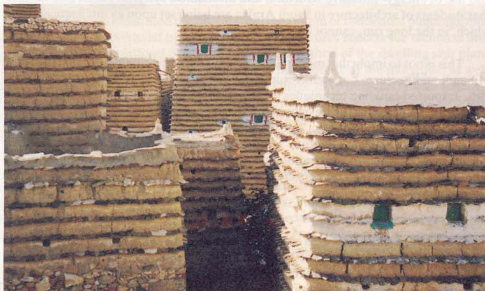
Fig. 15. Crowded houses arrangement provides shading and reduces the areas exposed to the Sun.
