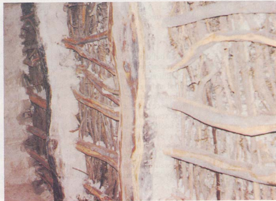
Fig. 10. a. Interior view towards the ceiling. b. Cross section in partially collapsed building showing roofing system details.
