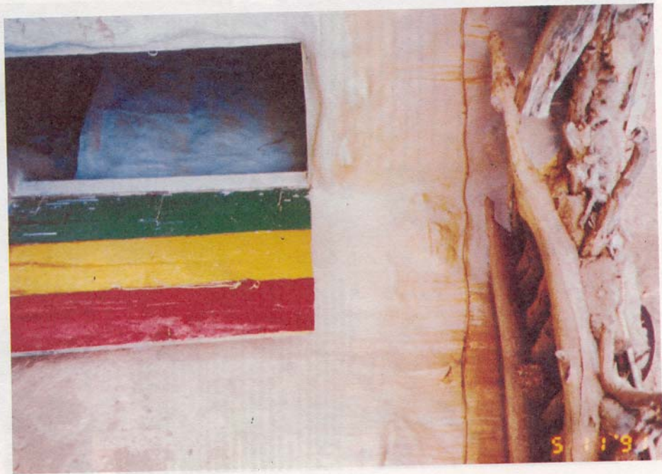
Fig. 9. Wooden beams (tree trunks) are used to support floors, roofs and stairflights. (See also Fig. 14)
