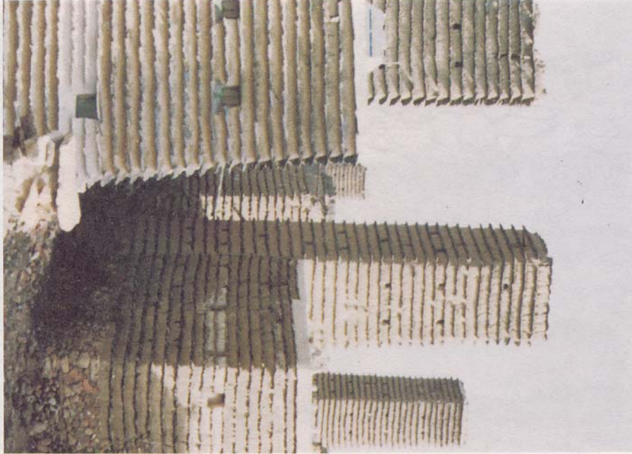
Fig. 5. Raqaf (slate) stone courses are built in alternate courses with mud courses. Buildings are shaped conically towards the roof for structural purposes.
