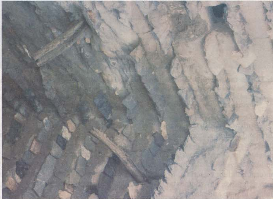
Fig. 13. a. Wooden gutters are used to facilitate rain water drainage. b. A Hall is built under the main entrance sill to drainout rain water collected in the fima (Yard) space.
