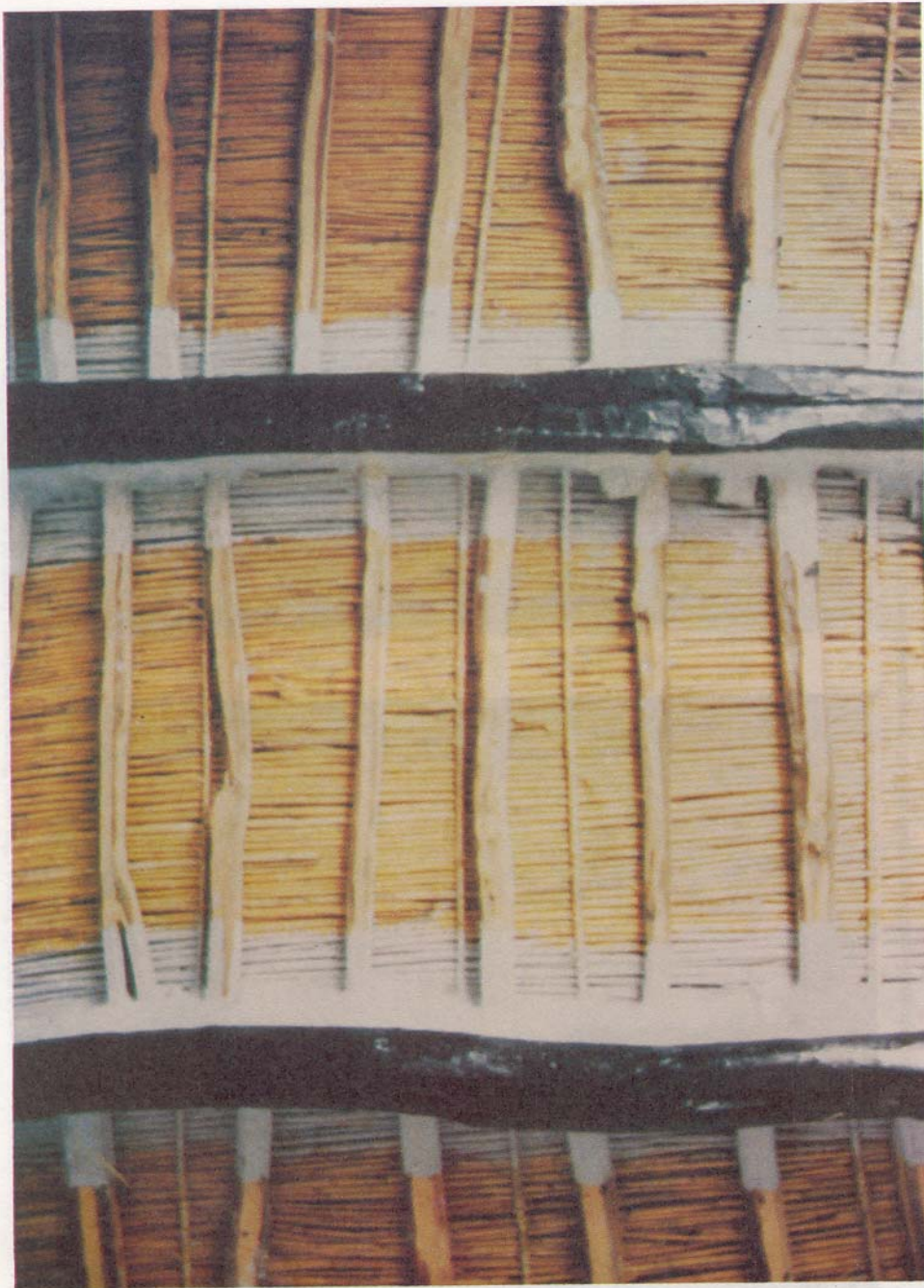
Fig. 12. Interior view showing the use of Sorghum stems in spanning narrow spaces.
