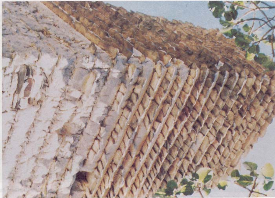
Fig. 5. Raqaf (slate) stone courses are built in alternate courses with mud courses. Buildings are shaped conically towards the roof for structural purposes.
