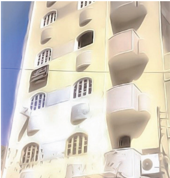
Figure 13. Balconies & Low window ratio.
