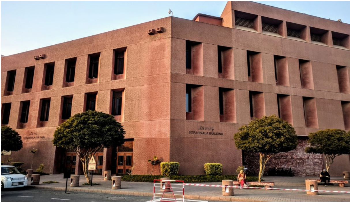
Figure (3). The AKUH, which is one of the case studies, and is cited by Abel (1994) as an example of a Critical Regionalist project within Karachi
