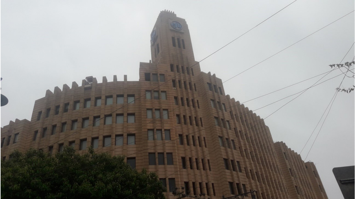
Figure (1). Qamar House in Karachi constructed between 1946 and 1955 by Qamardin & Co is an example of experimentation of core built form in search of an identity for the newly independent city/ country
