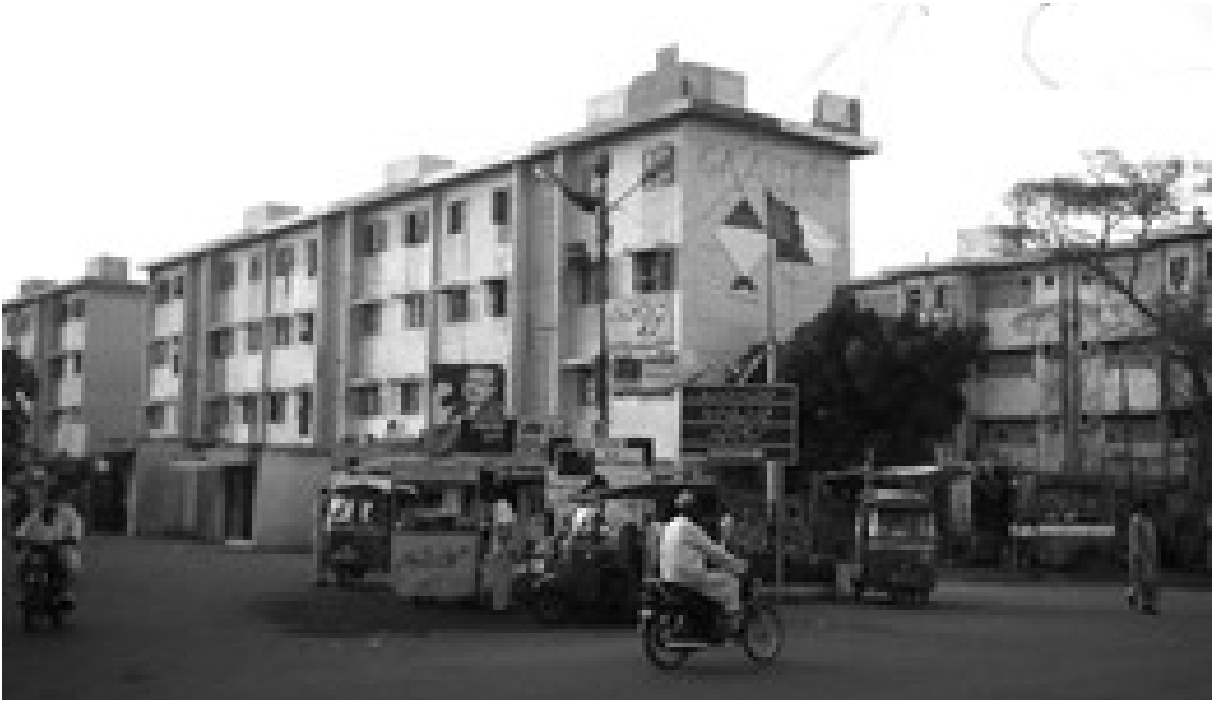
Figure (5). An example of sprawling built form in Karachi
